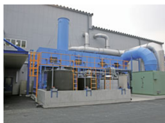
▲薬液洗浄装置 Chemical cleaning equipment
