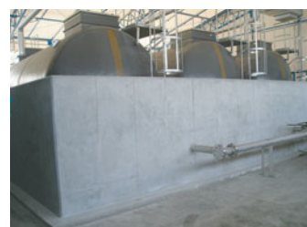
▲防液堤(RMC) Bank for leakage (RMC)
