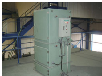
▲脱臭装置 Deodorizing equipment
