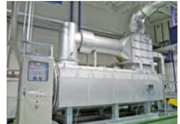
▲脱臭炉 Deodorizing furnace
