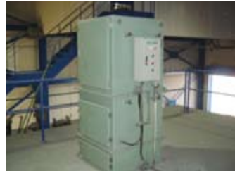
▲脱臭装置 Deodorizing equipment
