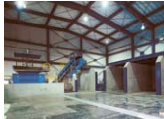
▲鉄板を敷いた床面 The floor covered with iron plate
