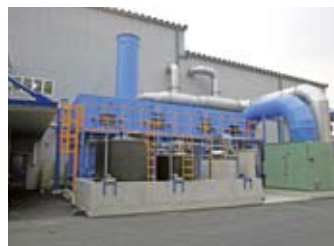
▲薬液洗浄装置 Chemical cleaning equipment
