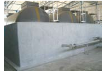
▲防液堤(RMC) Bank for leakage (RMC)
